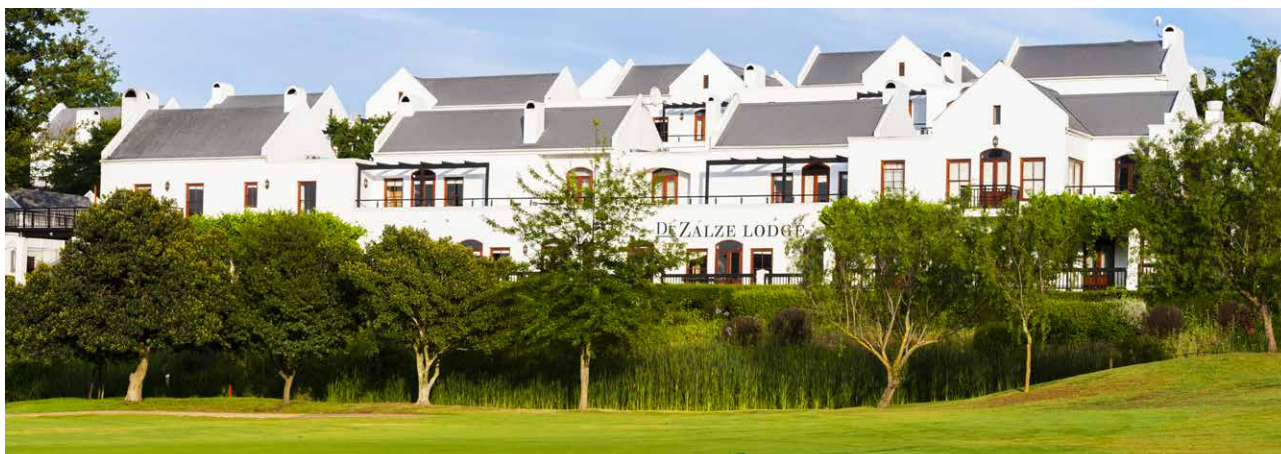
De Zalze Lodge, Stellenbosch, South Africa 33 58'13.66" 18 50'09.55" E
